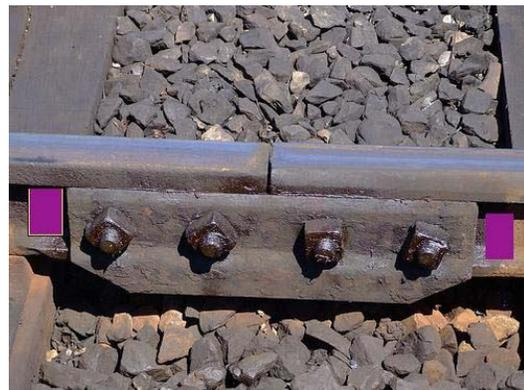
Fig 1. A Fish Plate with suitable position of sensors
